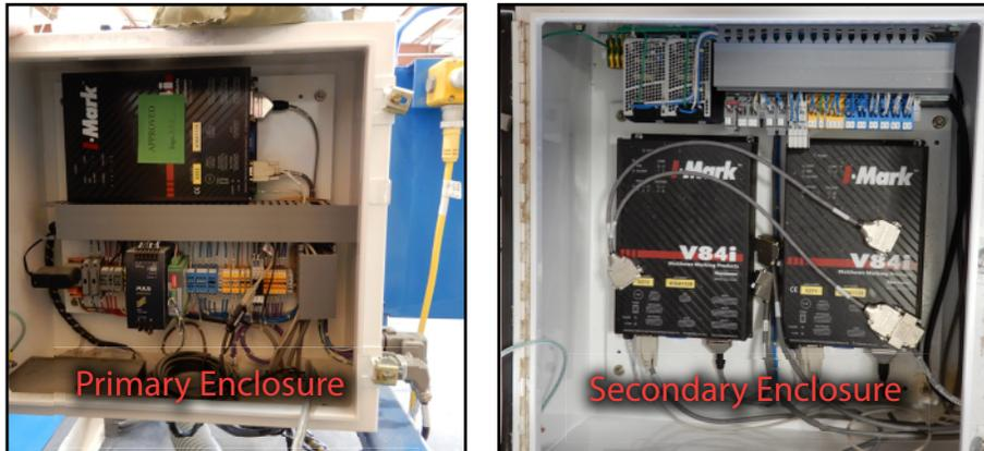
3. In the V84i primary enclosure, disconnect the **Gripper** (top rearmost) and **LASM** (bottom rearmost) encoder cables. Before proceeding to next step, mark the connectors as Gripper and LASM (see Figure 3).
