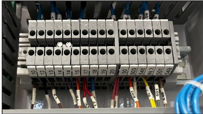
14. From the 20-ft cable, connect the brown wire to the terminal block 14 bottom.
