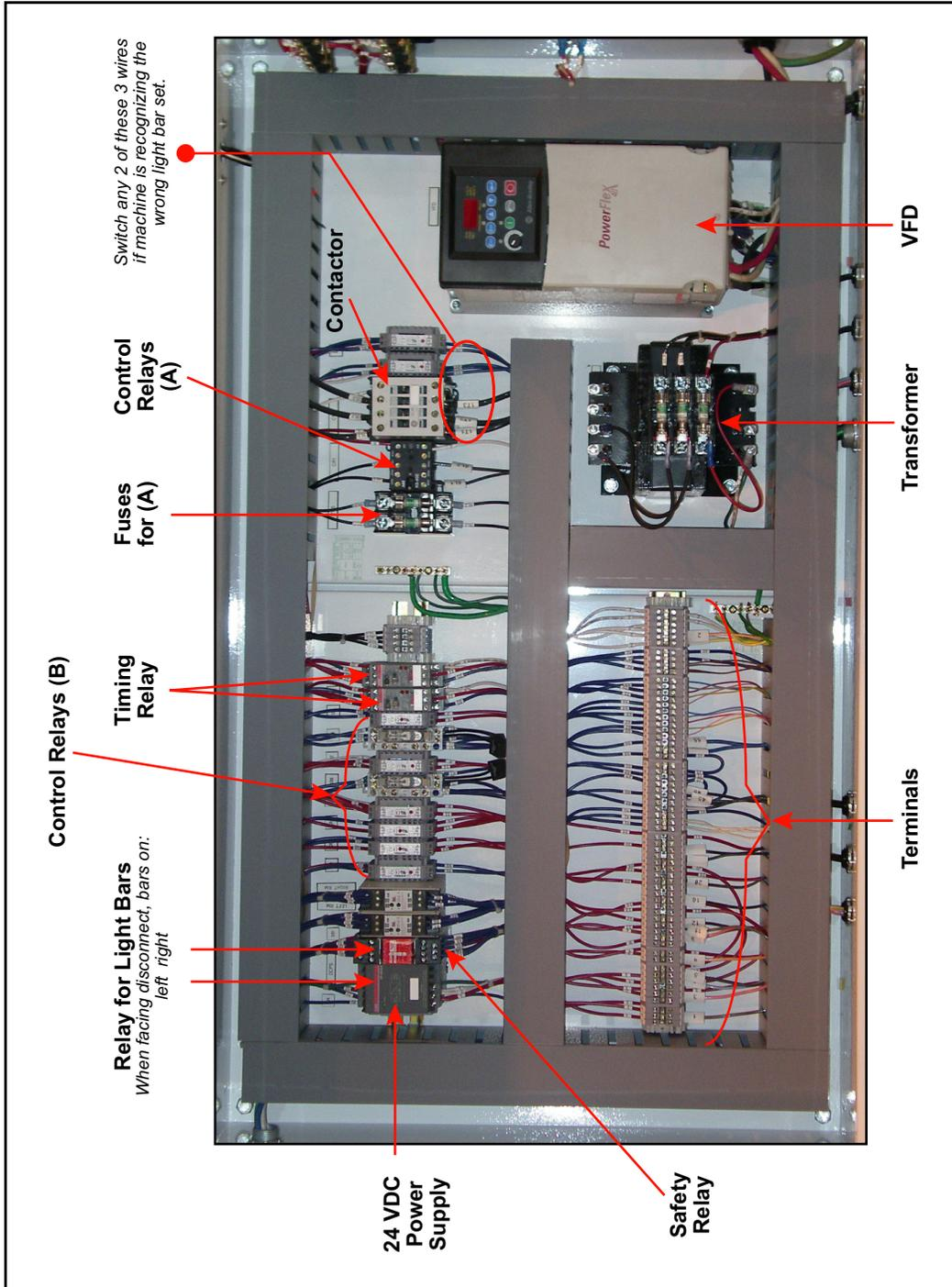
Figure 6-31: Electrical Enclosures for a 2-Enclosure System
