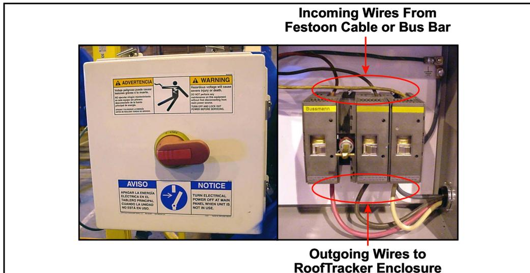
Power is brought into the disconnect enclosure and connected to the terminals on top of the fuses. The wires are labeled *Incoming Wires From Festoon Cable or Bus Bar* in Figure 3-4. The order in which they are connected is irrelevant because you will perform a test later and switch the wires at the VFD if the direction of travel is incorrect. Refer to your electrical schematic for detailed wiring instructions.
