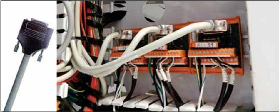
5. Tighten the screws on the interface module end of the PAC.
