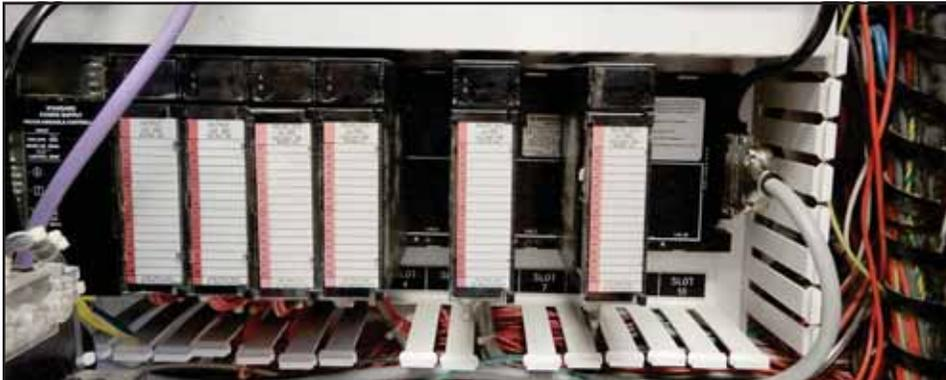
**Figure 20: Carriage-End Output Modules Removed**
