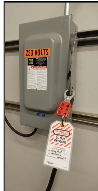
Figure 1: Lockout/Tagout on the Power Source Panel
