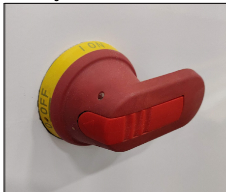
Figure 1: Disconnect Switch
